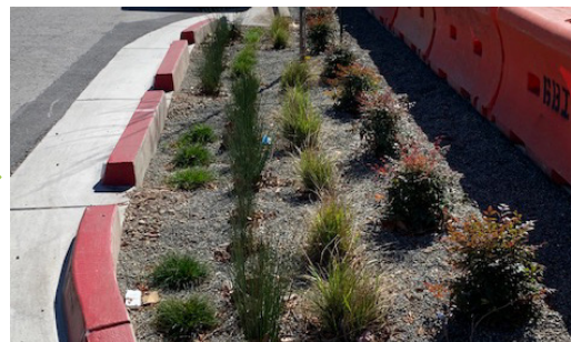
Bioswales filter pollutants
